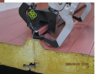
**Step #3**- Remove the hand crimper and clamp. Crimp once again at the end of the run to form the small "tag" remaining from the clamped area.
