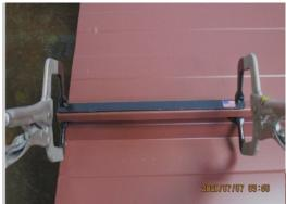
Note: There should be "foam-to-foam" contact on each adjoining panel.
